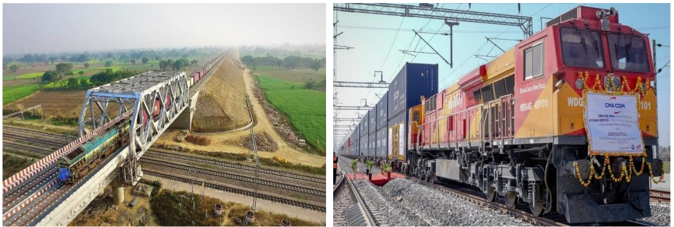
Dedicated Freight Corridor (DFC)
